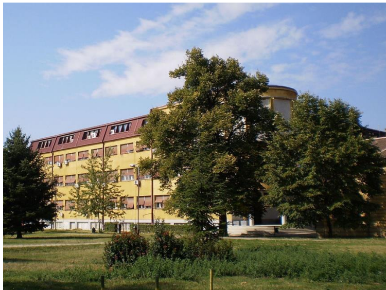
1. Public Health Institute Niš - view from the east
